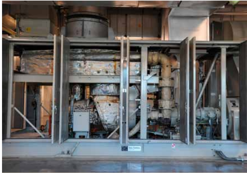
The combustion turbine is the heart of a CHP plant.
